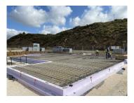
Eco Building Group uses an insulating formwork that ensures a strong connection to the walls without thermal bridges.
