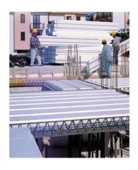
Panels are originally self-standing, that is they can stand any weight (concrete casting, workers, reinforcement steel, etc.) with traditional and simple shoring system with prop supports at a maximum distance up to 2 meters.
