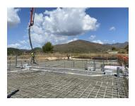
Reinforcement and spacers, that are suitable for insulation on soft surface, are being placed to make sure that there is sufficient concrete cover.
