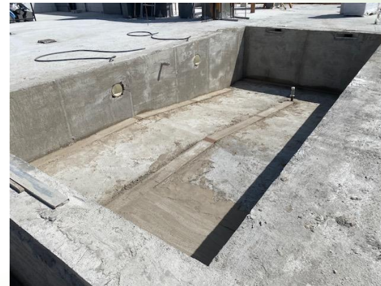
Rough pool level before waterproofing layer
