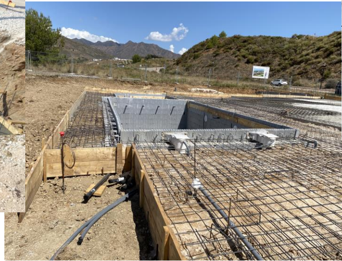
Finished pool walls and reinforcement surrounding terraces
