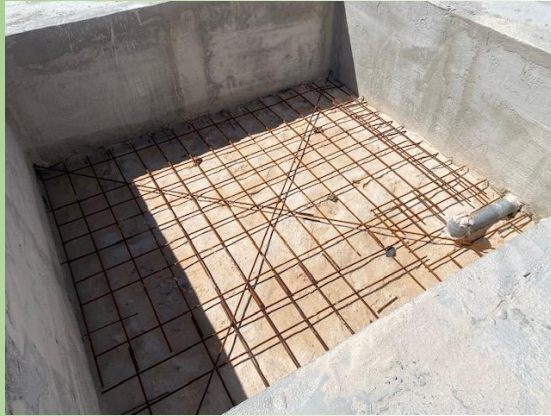
Reinforcement chill out
