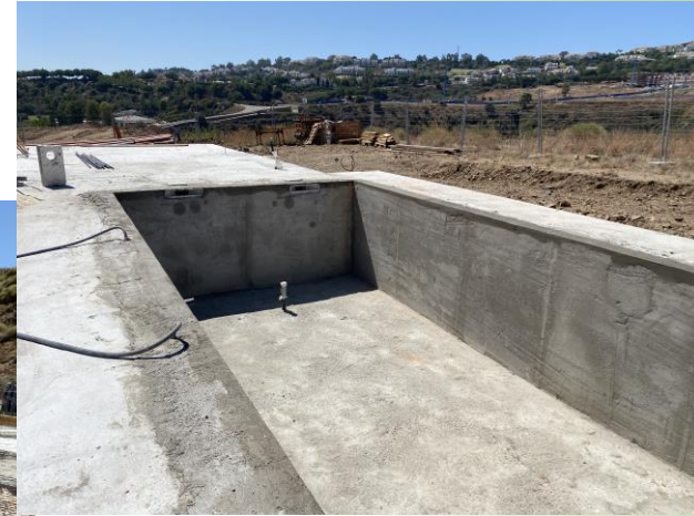
Rough construction finished
