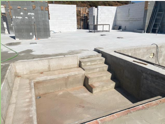
Seats and steps rough works chill out before waterproofing
